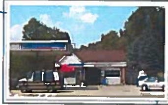
Leaking UST Releases
