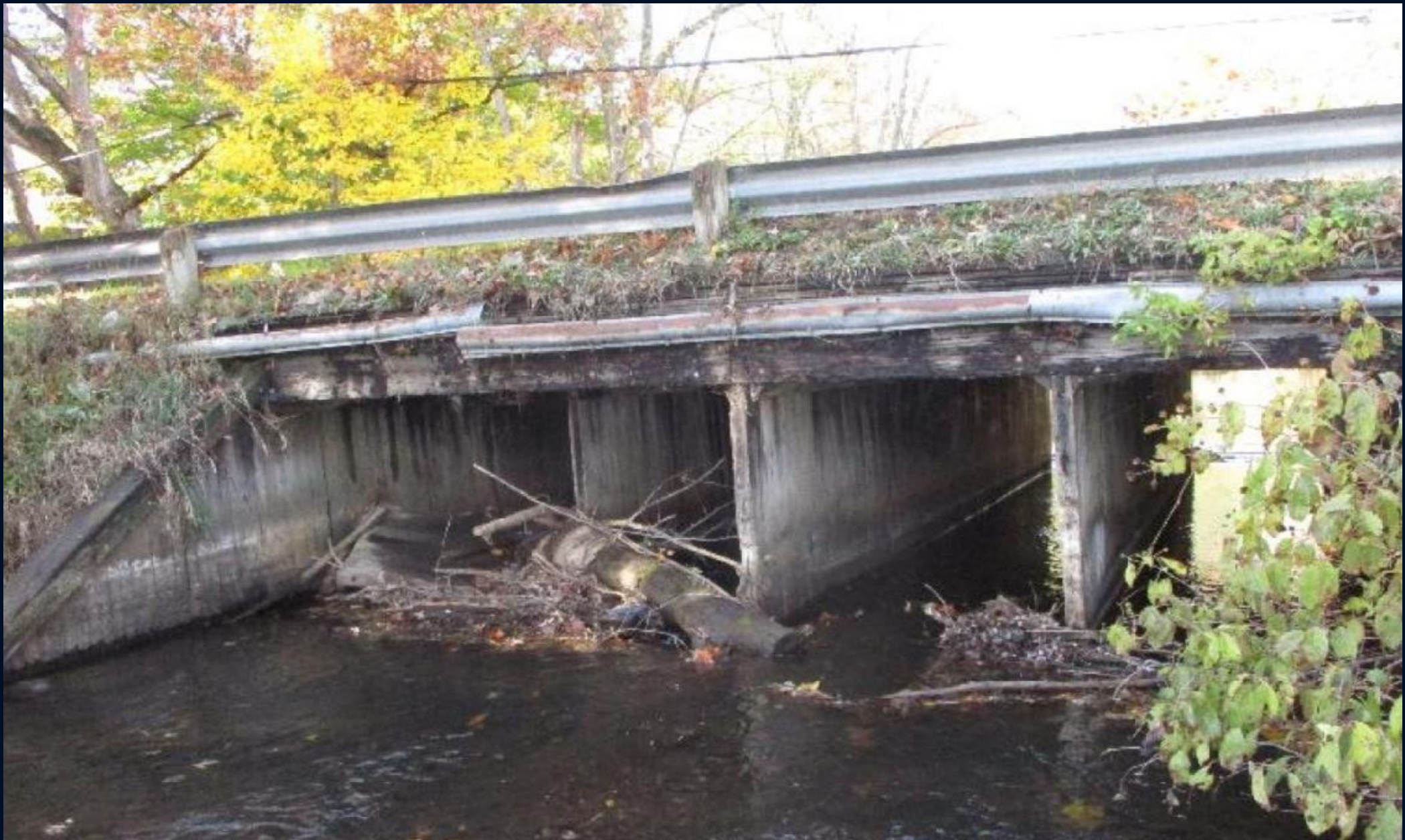
Branch County - Fiske Road
