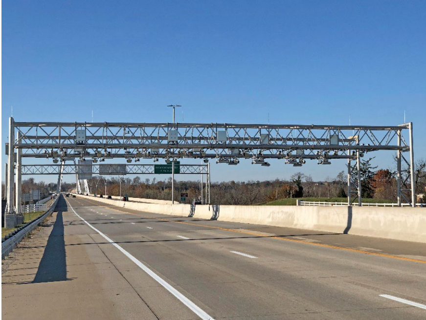
All-electronic toll gantry on the East End Crossing toll bridge over the Ohio River between Indiana and Kentucky
