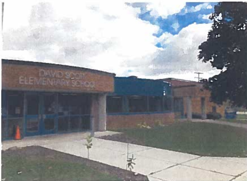
David Scott Elementary School in DeWitt. State environmental regulators fined a contractor overseeing renovations $15,000 for an asbestos release. (Photo: Craig Lyons)
