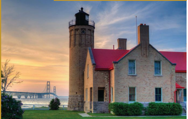
Old Mackinac Point Lighthouse (Mackinaw City)
