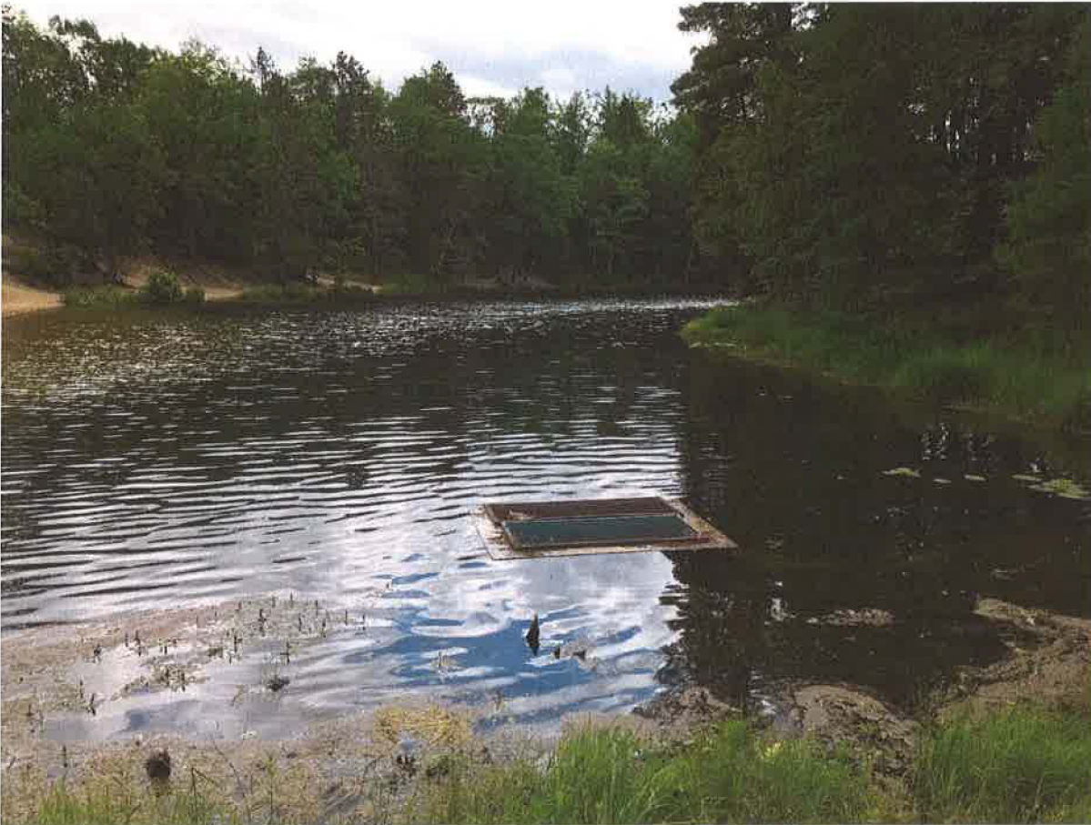
Figure 3. Example of an uncontrolled spillway with a fixed crest.
