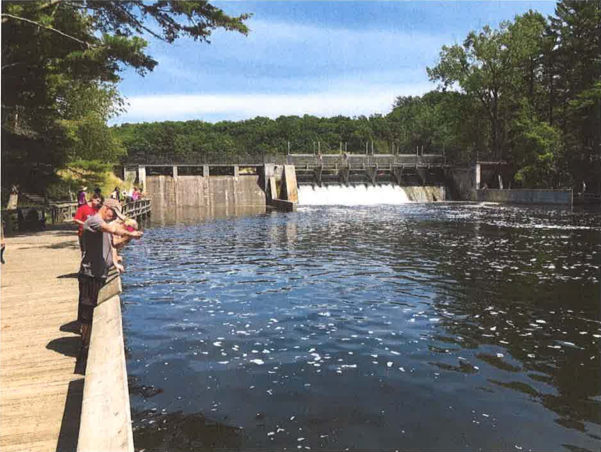
Figure 2. Example of a controlled spillway with several gates.
